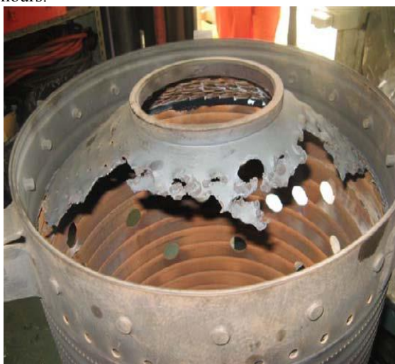
Figure 23 – ABK PGT10 2-Shaft Combustion Liner Subject to Hot Corrosion after 8,000 Running Hours with Low Grade Air Filtration –
