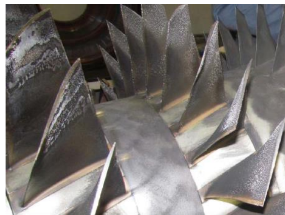
Figure 18 - ABK SGT400 Compressor Fouling after 4000 Running Hours with the initial M5 Filtration Grade -
