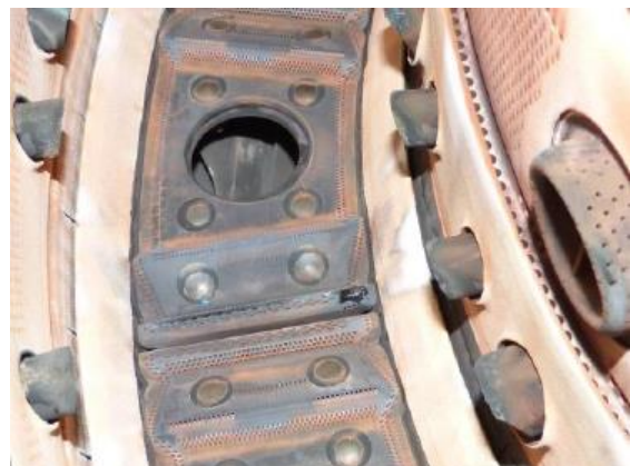
Figure 25 - ABK RB 211 Front Combustion Liner Re-Usable after 7650 Running Hours and E12 High Grade Filtration -
